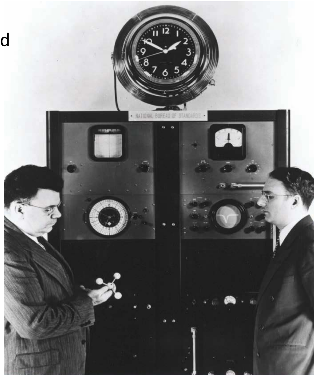
Figure 5. The first atomic frequency standard, based on the ammonia molecule (1949). Inventor Harold Lyons is on the right; Edward Condon, then the director of NBS, is on the left.
